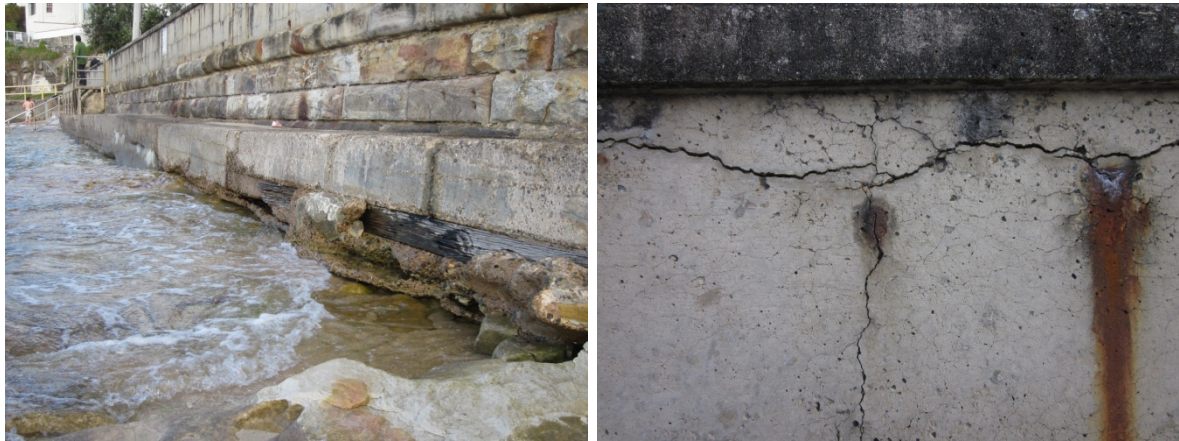
Figure 3.5 Fairy Bower Seawall Photos of Present Condition
