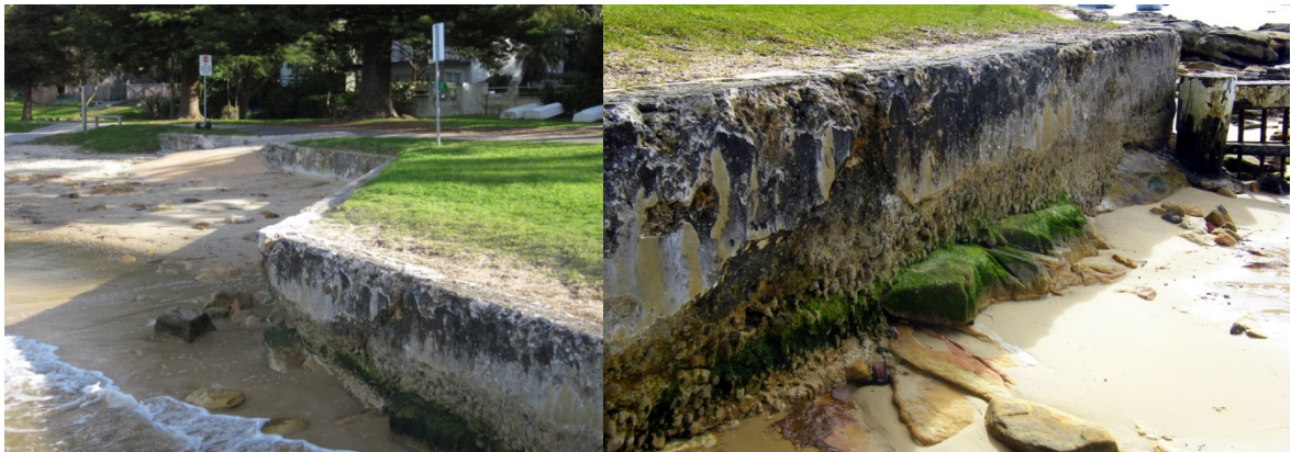
Figure 3.3 Forty Baskets Seawall Photos of Present Condition
