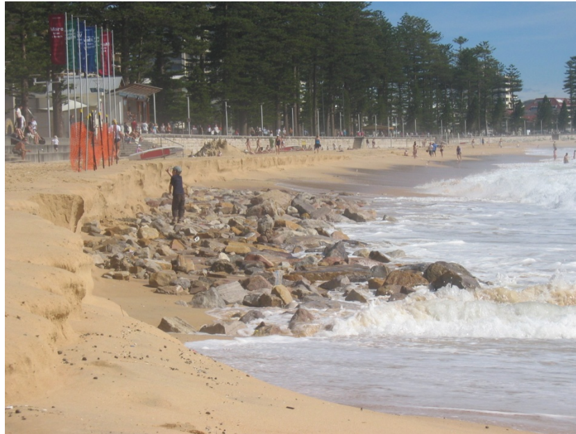
Figure 4.7 Photo of Eroded Beach near Manly LSC (06/02/2008)
