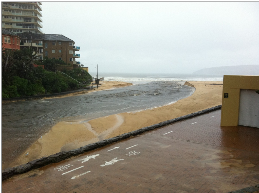
Figure 6-5 Scoured entrance during March 2011 event (Source: MHL)
