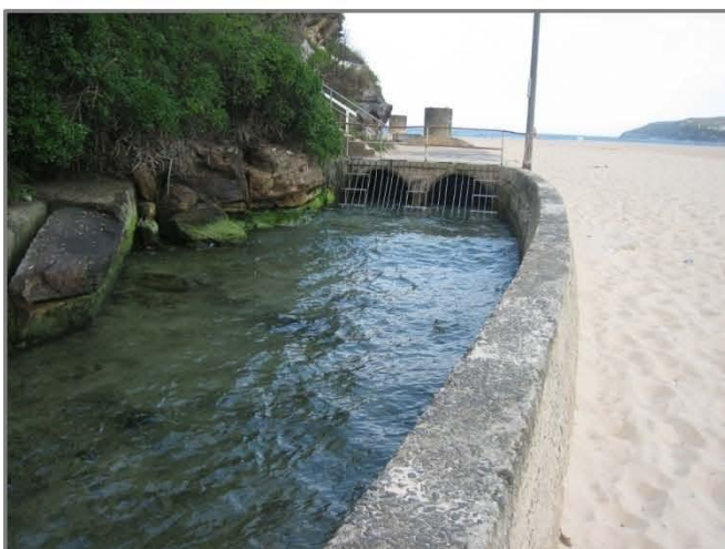
Low-flow pipes at channel entrance
