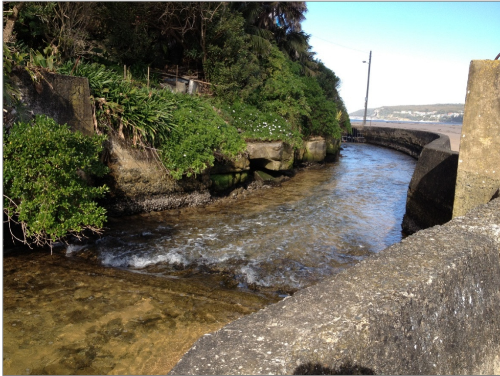
Figure 6-4 Manly Lagoon concrete entrance channel
