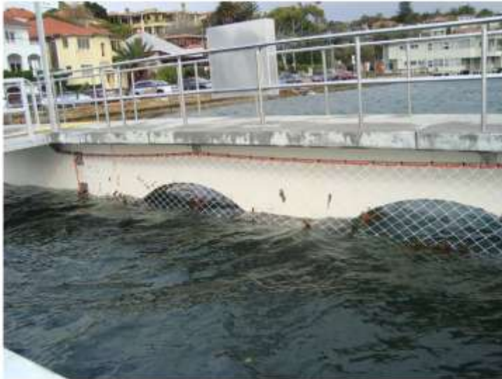
Photograph 2. Trampoline style nets showing net and steel cable detail. Note the limited vegetative growth one year after installation: The nets mistakenly had anti-fouling on them.
